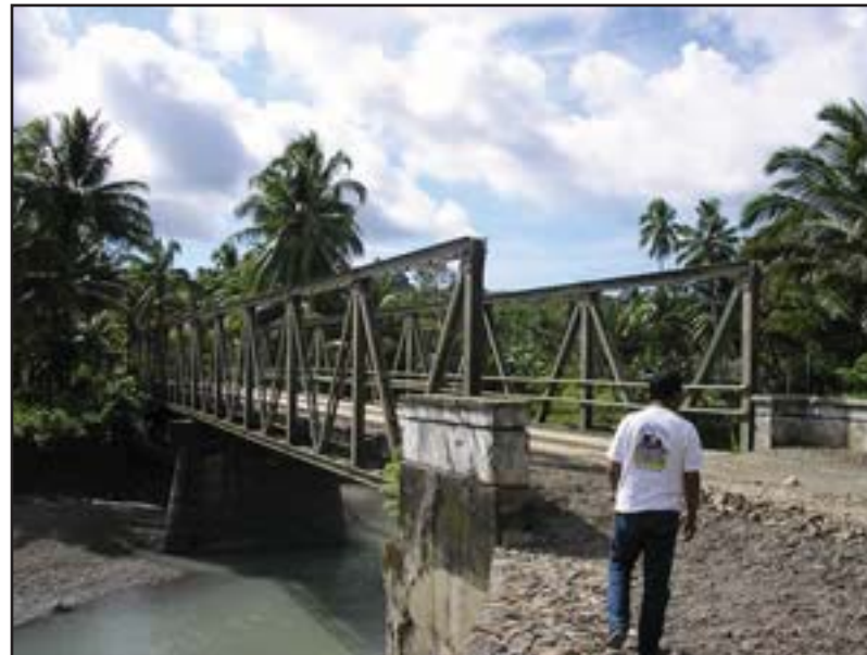
GIS was an invaluable tool in planning the infrastructure repair work.
