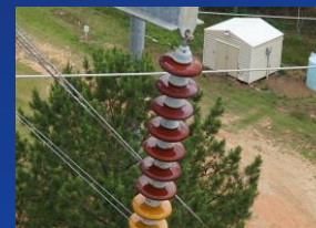
Drone close range inspection
